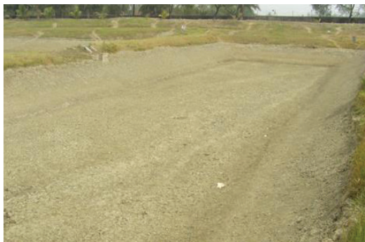
Pond bottom after top soil removal
