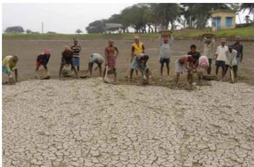
Top soil removal
