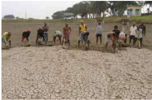
Top soil removal
