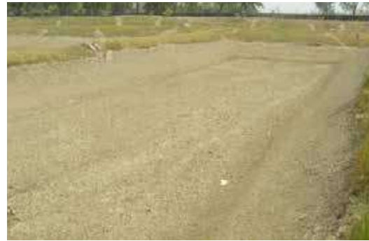
Pond bottom after top soil removal
