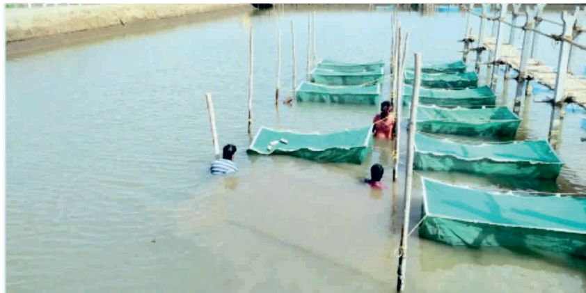
Bamboo installation and hapa fixation
